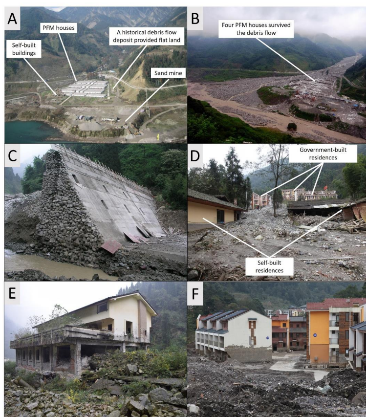
Figure 10: Losses caused by the Aug 14, 2010 debris flows. The locations of the examples are shown in Figure 8. A: The temporary settlement at the Bayi sub-catchment outlet in 2009 (Luo et al., 2010); B: The shelters destroyed by a debris flow from the Bayi sub-catchment (Luo et al., 2010); C: One of the two under designed check dams in Bayi sub-catchment which were destroyed (Liu, 2010); D: Residences reconstructed on old debris flow deposits were damaged; E: A hotel beside the Longxi River was struck; F: government-built apartment buildings beside the river were damaged.
