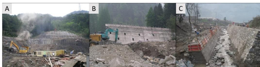
Figure 7: Mitigation works that were under construction in 2010. A: stabilized slope near the newly built primary school in Longchi town. B: check dam being built in the Bayi sub-catchment after a debris flow in 2009. C: drainage channel being built at the outlet of the Bayi catchment after the debris flow in 2009.
