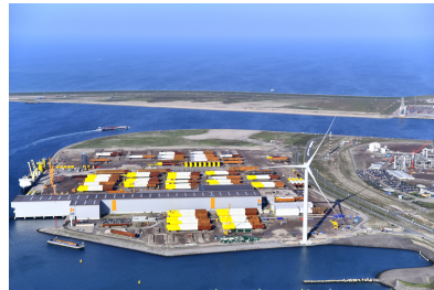
(b) The 12\text{MW} GE Haliade X at the port of Rotterdam [3].
