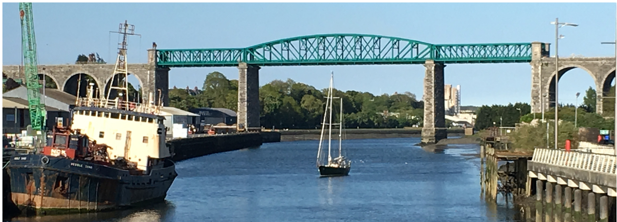
Figure 2: The Boyne viaduct railway bridge in Drogheda, Ireland.
