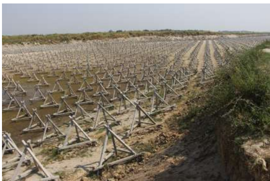
Figure 1: Porcupine field in secondary channel of Ayeyarwady River, Myanmar. Photo courtesy of H. Fredrikze, Royal HaskoningDHV.
