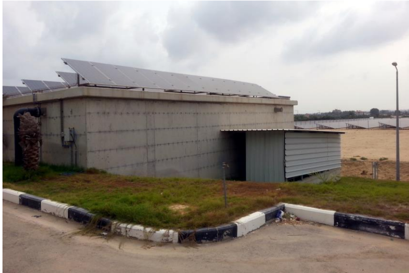
Figure 4. Photovoltaic panels at the Southern Gaza Desalination Plant. Photo credits: Juliane Schillinger, October 2018.
