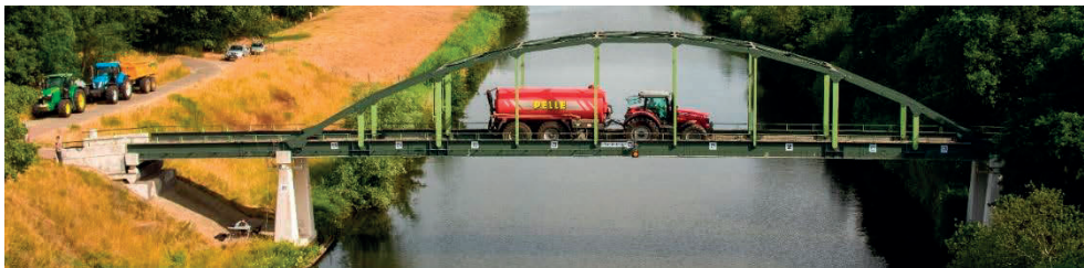
Figure A.1 Tankinkbrug with proof loading vehicle.
