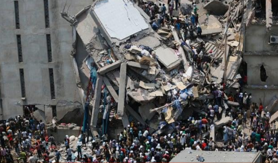
Rana Plaza Collapse Source: The Guardian
