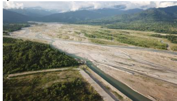
Figure 1. Potential area for land reclamation in the Mao River.
