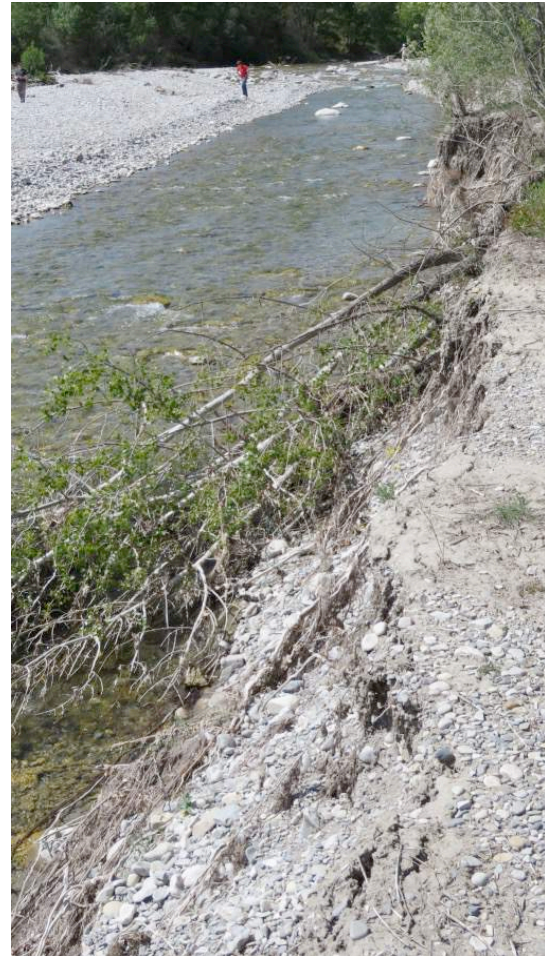
Figure 2. Areas of active bank erosion illustrated by the tumbling trees. At these locations the erosion between 2014 and 2015 was measured using DGPS and used as reference for UAV image assessment of bank erosion.
