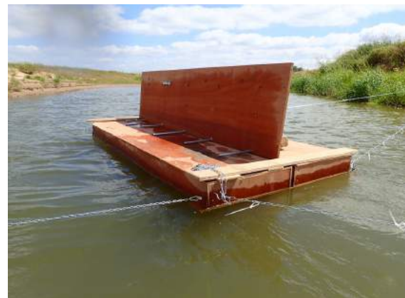
Figure 1. Surface screen mounted between two barges and attached to the banks using chains.
