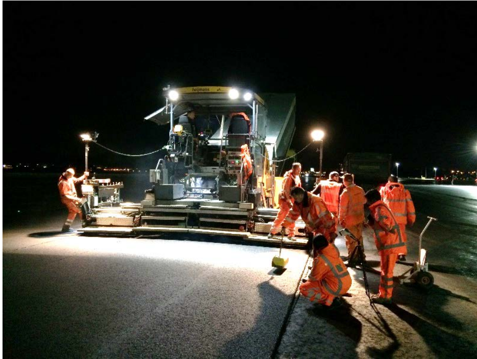
Figure 7 - Picture while measuring the density after the paver on-site.
