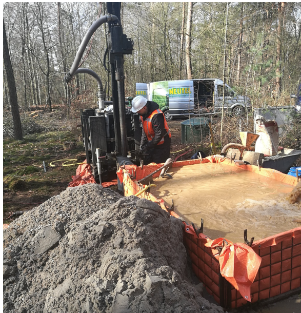
Figure 2. Drilling of boreholes for FBG fibers and piezometer.
