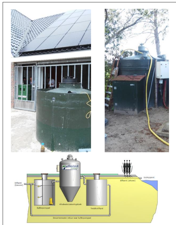
Figure 4.1 a) Schematic process flow diagram and pictures of installed prototype MBR setup in Delft-the Netherlands b) Decentralized wastewater treatment system Bever III from the company Afmitex in Friesland the Netherlands.
