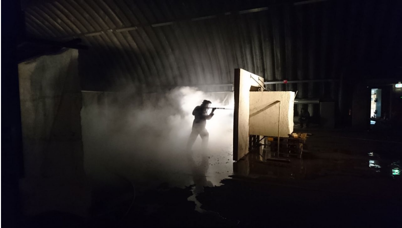
Figure 26: Material playground. Exploring the possibilities of hydro-demolition for Luftschluss.
