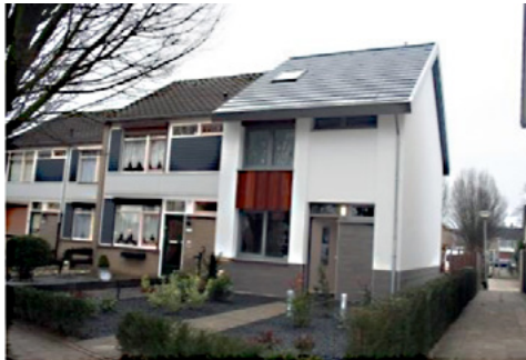
Figure 1: Kerkrade, where passive cooling measures were applied in the shape of an overhang, night ventilation grid and improved insulation
