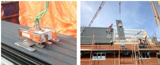
Figure 3: Roofing sheets were lifted piece by piece (Berben, 2015)
