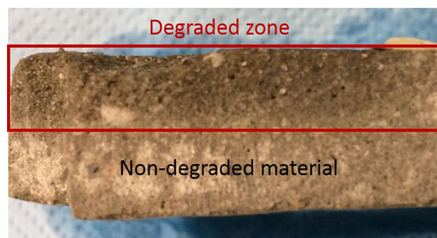
Fig. 2 Leaching of calcium in cementitious material. Transition between pristine and degraded material is composed of gradual layers of calcium content (Color figure online)
