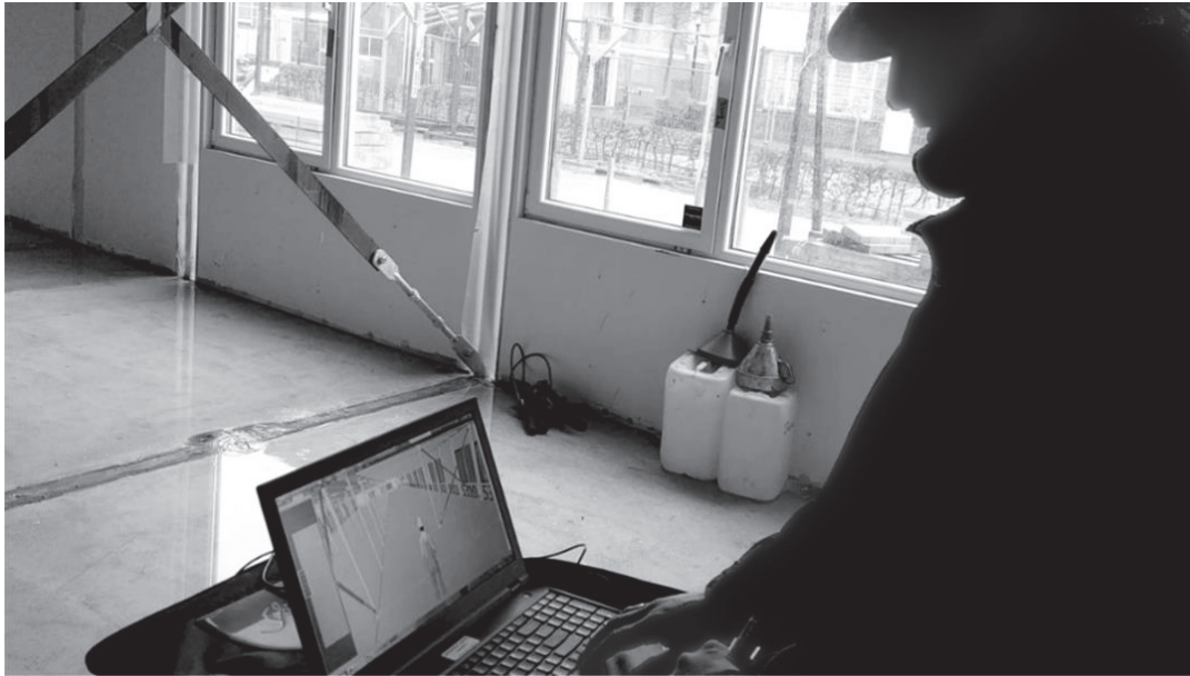
Figure 1: Overview of new routine - on-site use of a virtual environment for tagging elements
