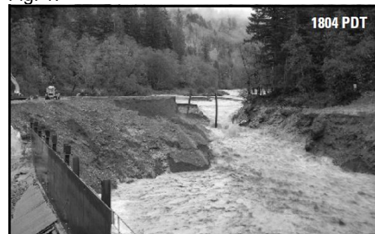
Figure 1. Breaching of the Cofferdam and initiation of Reservoir Erosion, 19 Oct. 2007, (Major et al., 2012)
