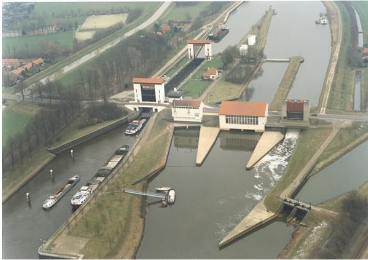
Figure 15. The canal lock (left hand side) and the water pumping station, source: RWS.
