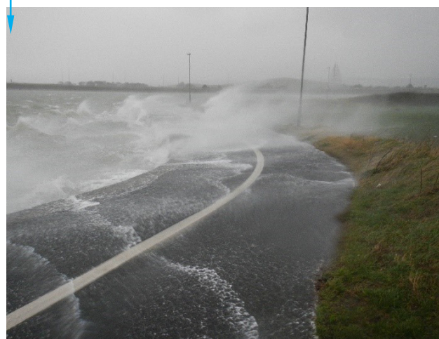
FIG. 1 Wave overtopping on a dike with a road on top of the dike crest resulting in roughness transitions.
