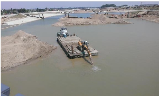
Figure 1. Excavation of flood channel along river Waal at Nijmegen under the Room-for-the-River programme.
