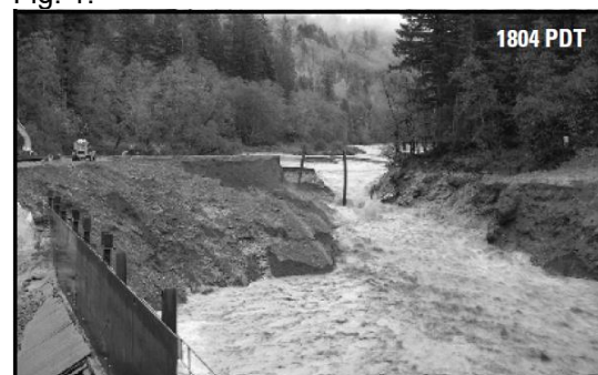
Figure 1. Breaching of the Cofferdam and initiation of Reservoir Erosion, 19 Oct. 2007, (Major et al., 2012)
