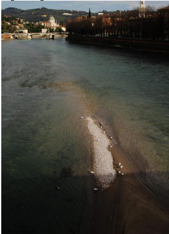
Figure 1. Forced bar near the downstream face of a bridge pier in River Adige, Verona, Italy.
