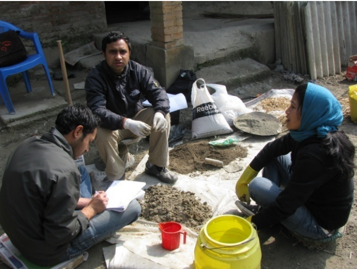
Fig: Mixing material
