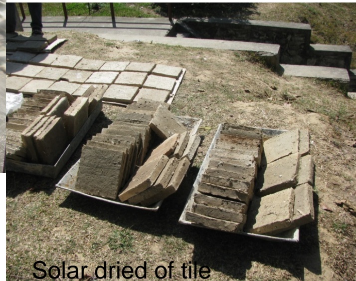
Fig: Preparation of Insulation tile
