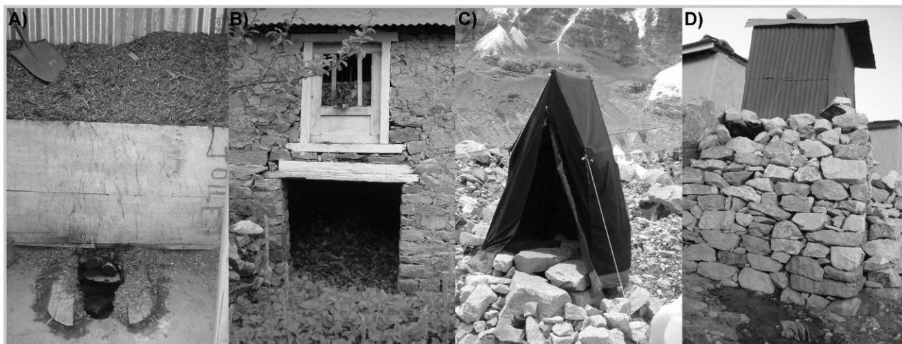
FIGURE 4 Types of toilets in SNPBZ. From left to right: (A) and (B) 2 toilets using litter, the most common type of toilet in the lower part of the park; (C) a temporary toilet at Everest Base Camp; (D) the toilet of a hotel showing waste flowing out on the surface from a septic tank. (Photos by Pramod Kumar Jha, Bharat Babu Shrestha, and Narayan Prasad Ghimire)
