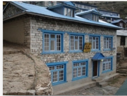
Fig. 2 Semi-modern building (Bhochhibhoya and Cavalli 2016)
