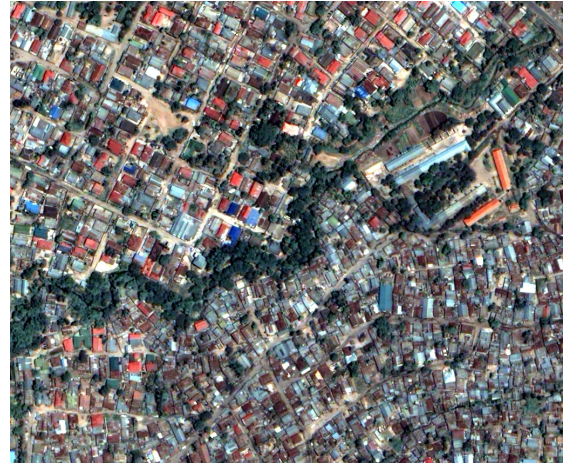
Fig. 1. Subset of the Quickbird data set considered in this letter illustrating different urban structures in Dar es Salaam: 1) formal urban area in the top and 2) an informal settlement in the bottom of the image.
