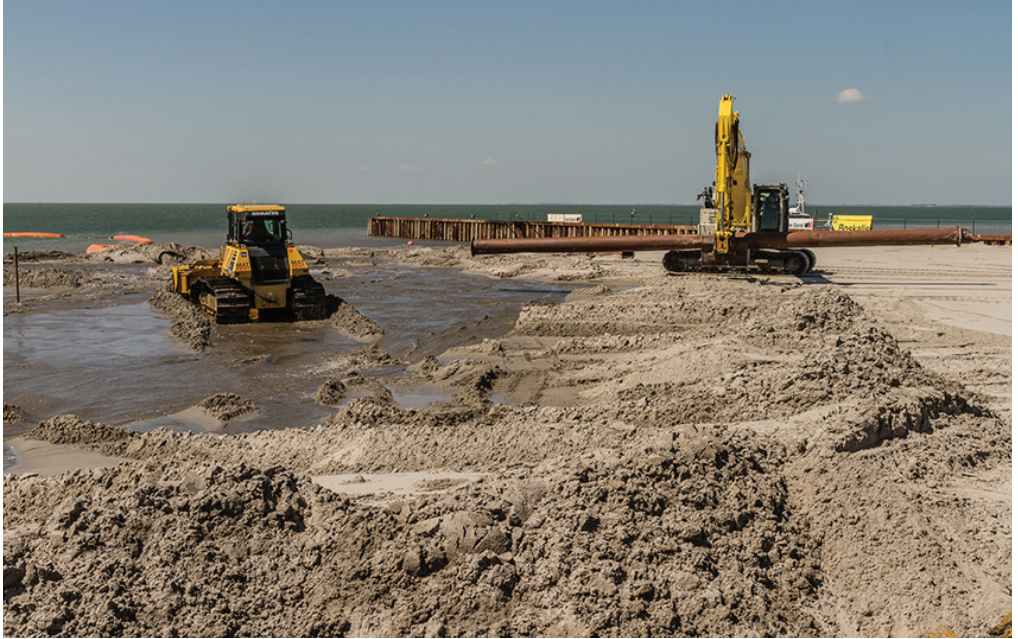
Figure 7.2 Work in progress at the Houtribdijk (Source: Rijkswaterstaat/ Harry van Reeken).
