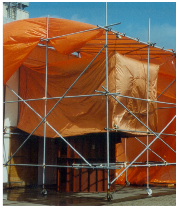
Figure 6: The VIRC as built for in-situ testing
