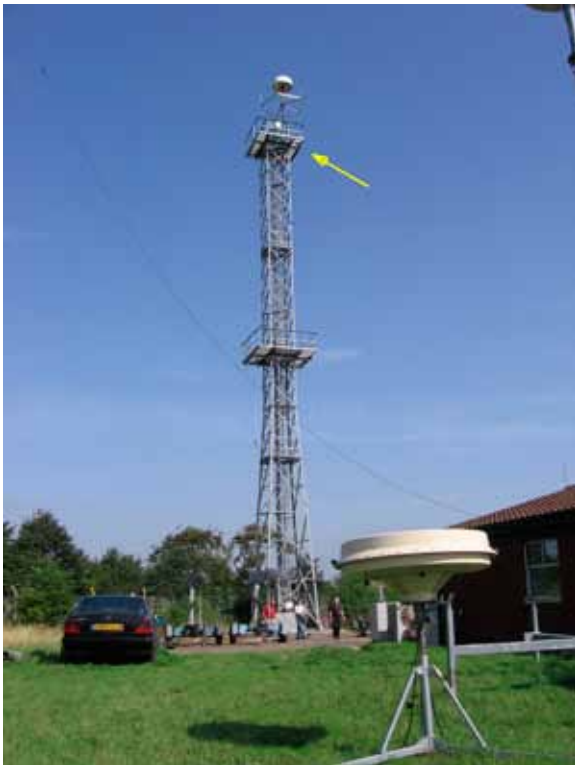
Figure 2-21: The antenna tower
