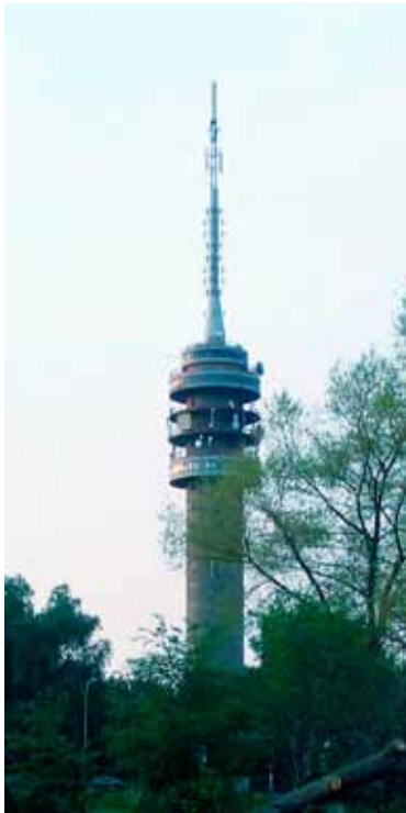
Figure 2-4: Goes antenna tower
