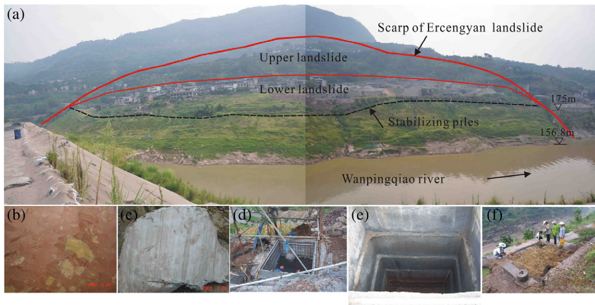
Fig. 2. (a) Photo of Ercengyan landslide and stabilizing piles; (b) Silty clay with gravels in the sliding soil (photo taken in 2002); (c) Striations on the slip surface from the shaft (2002); (d) Cast-in-place reinforced concrete piles (2006); (e) Reinforced concrete retaining wall inside pilehole (2006); (f) Top of a 3 \times 4.5 m rectangular pile (2007).
