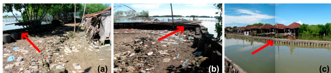
Figure 15. The embankment (shown by red arrows) for protecting the settlements (a–c). (c) shows the river and settlements built on the river banks prone to high tides from both the sea and the river.
