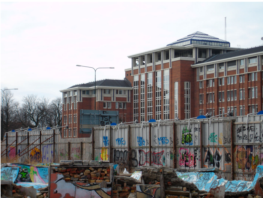
Figure 5. Co-existence of abandoned plots and active industries, Norra Sorgenfri, 2010.
