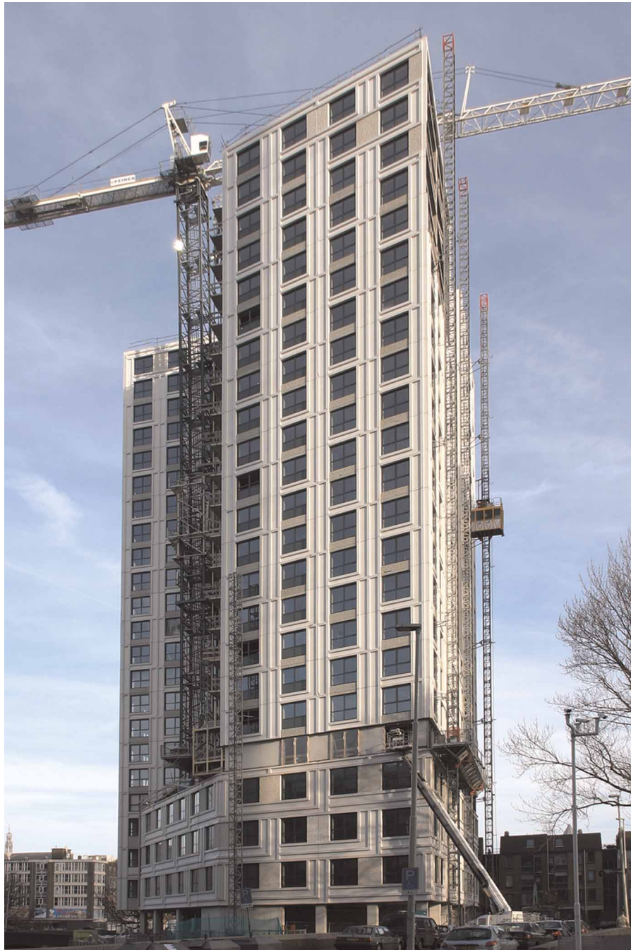
Figure 2 'Witte Keizer' project in Rotterdam under construction, 2004. Courtesy: http://www.skylinecity.info/
