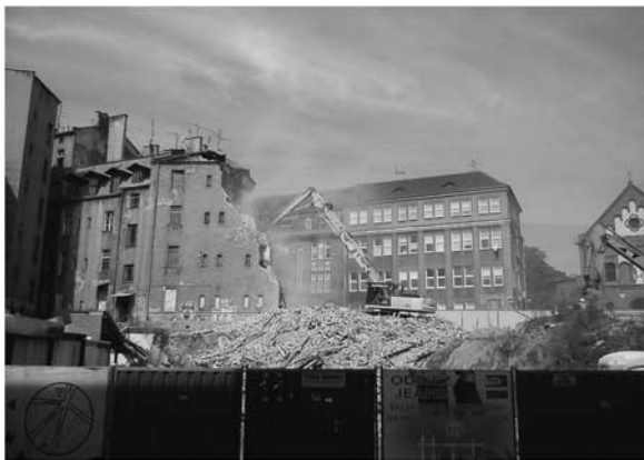
Figure 3: Planning for decline is an euphemism for demolishing buildings (picture: MOs810).
