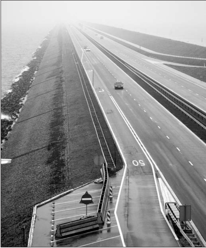
FIG. 1 The 32-kilometer-long Afsluitdijk, which closes off the Zuiderzee from the North Sea. To the right is the ocean, to the left the freshwater IJsselmeer. Due to a negative climate scenario, the entire dike will have to be raised nearly a meter in the next few years to meet the ten-thousand-year-flood standard. (Author's photo.)
