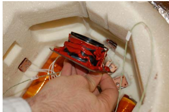
Figure 23. Installation of a DDRR antenna into the PU foam wall beneath the Fotino heatshield
