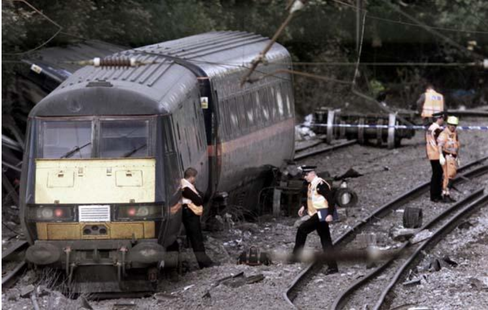
Figure 1.5 Hatfield derailment on 17 th of October 2000 because of broken rail due to Head Checks (photo Network Rail).
