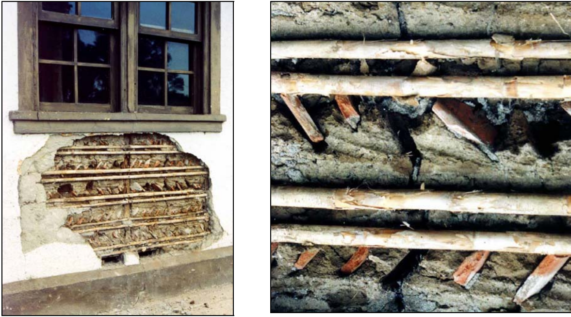
Figure 7.9: Typical Bahareque Wall
