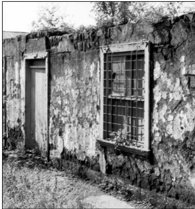
Figure 7.5: Typical Adobe Walls
