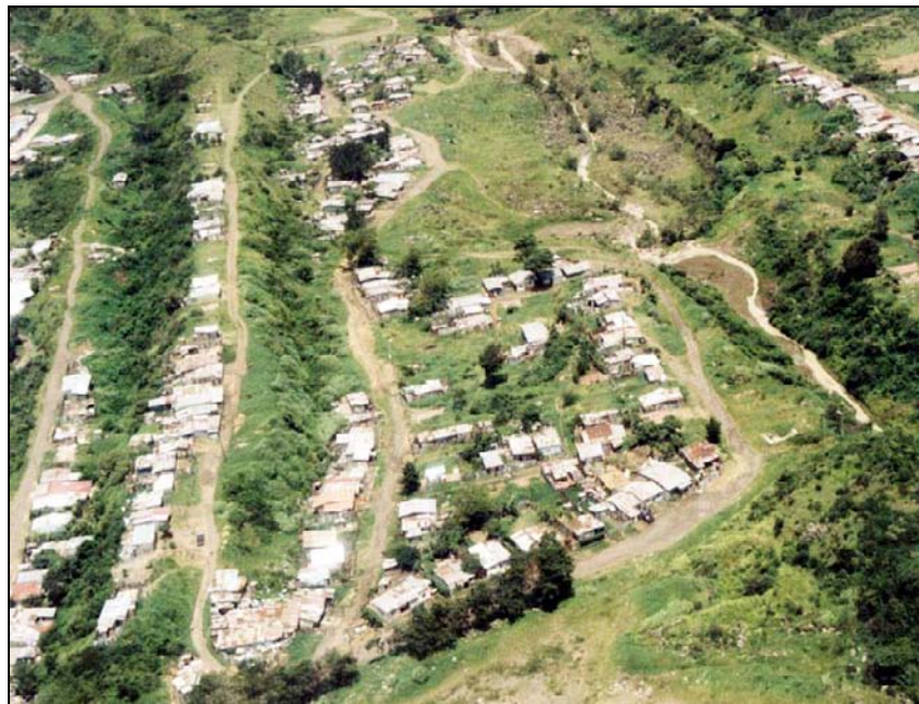
Figure 7.17: Squatter Occupation of the Floodplain inside the Perimeter of the Reventado River Dyke
