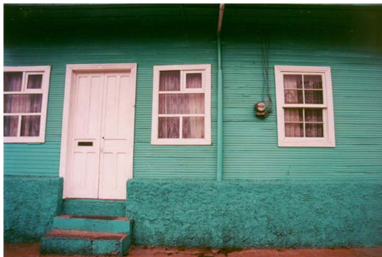
Figure 7.10: Mixed Adobe and Corrugated Metal Walls
