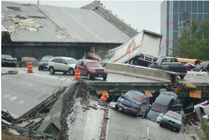
Figure 1.1. Bridge over the Mississippi river in Minneapolis, Collapsed Aug 1, 2007 [12]
