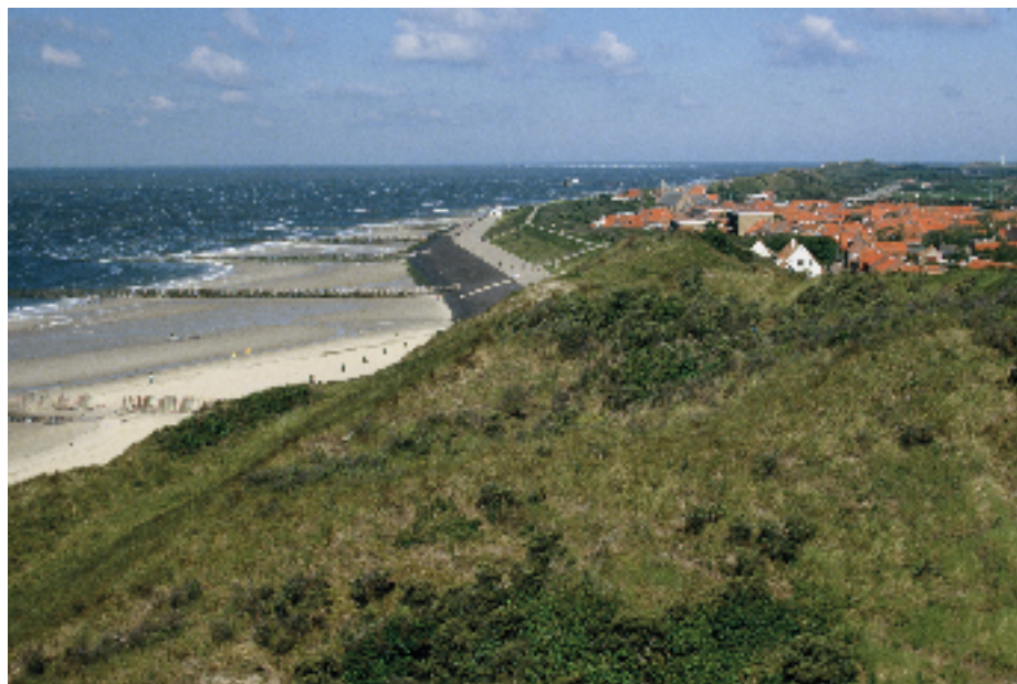
Figure 12.15 Hard and soft barriers along the coast. Westkapelle, small town in the province of Zeeland in the south west of the Netherlands, is protected by dikes and dunes. Source: Rijkswaterstaat, https://beeldbank.rws.nl
