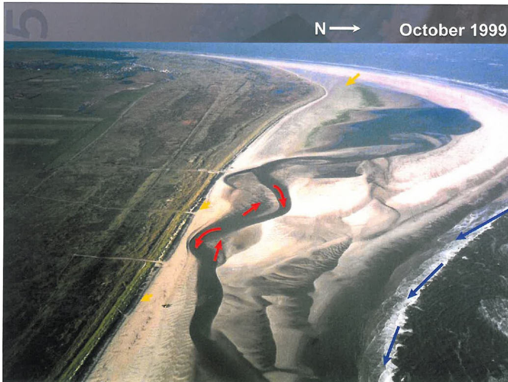
Figure 4: Erosion hotspots at the shoreline due to the formation of a meandering tidal channel at the Bornrif (Ameland, The Netherlands). Figure courtesy of Ministry of Public Works, Rijkswaterstaat (The Netherlands)
