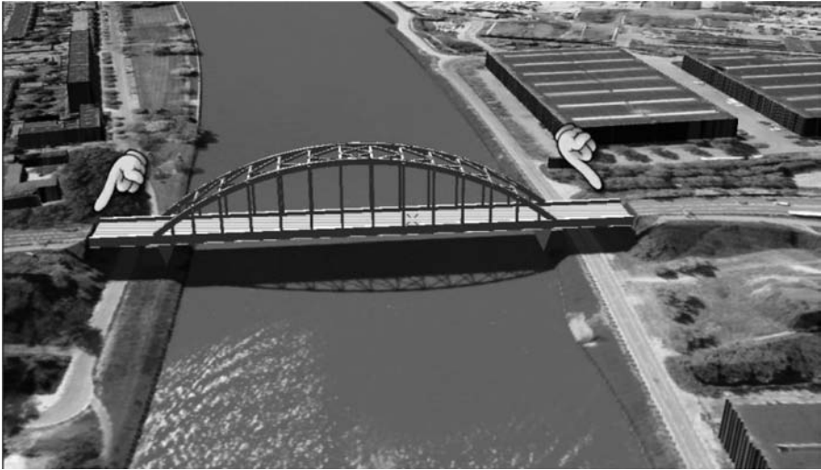
FIGURE 1.3 Bridge Amsterdam-Rijnkanaal near Utrecht. Courtesy of RWS/AGI.
