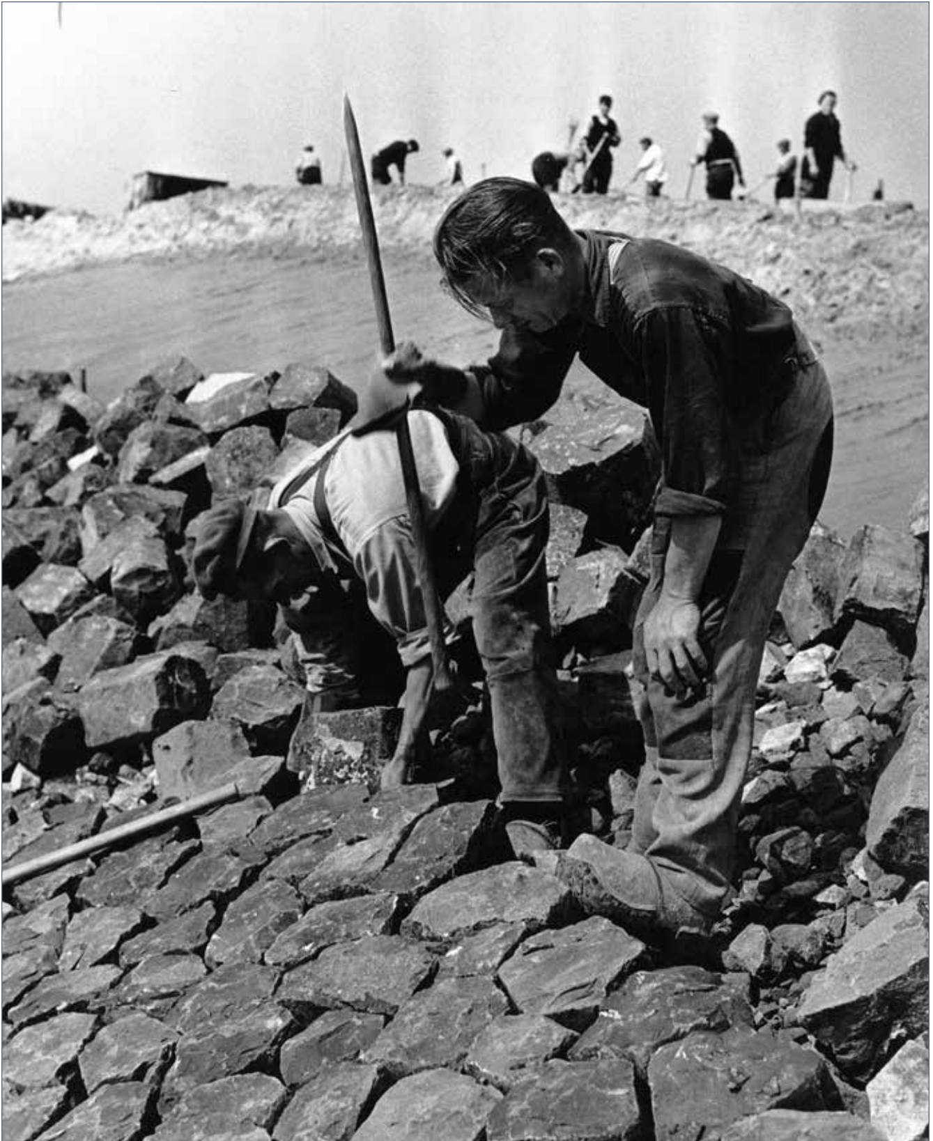
Stone-pitching in the dike surrounding Eastern Flevoland
