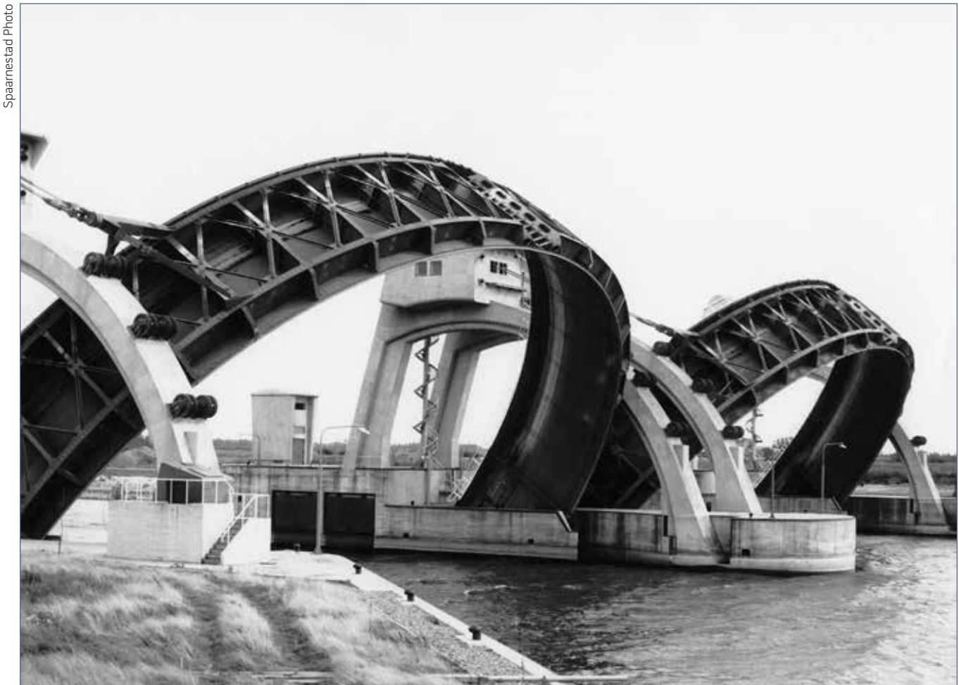
Weir at Hagestein, regulating the water level in the Nether Rhine during low stages to facilitate navigation, completed in 1958
