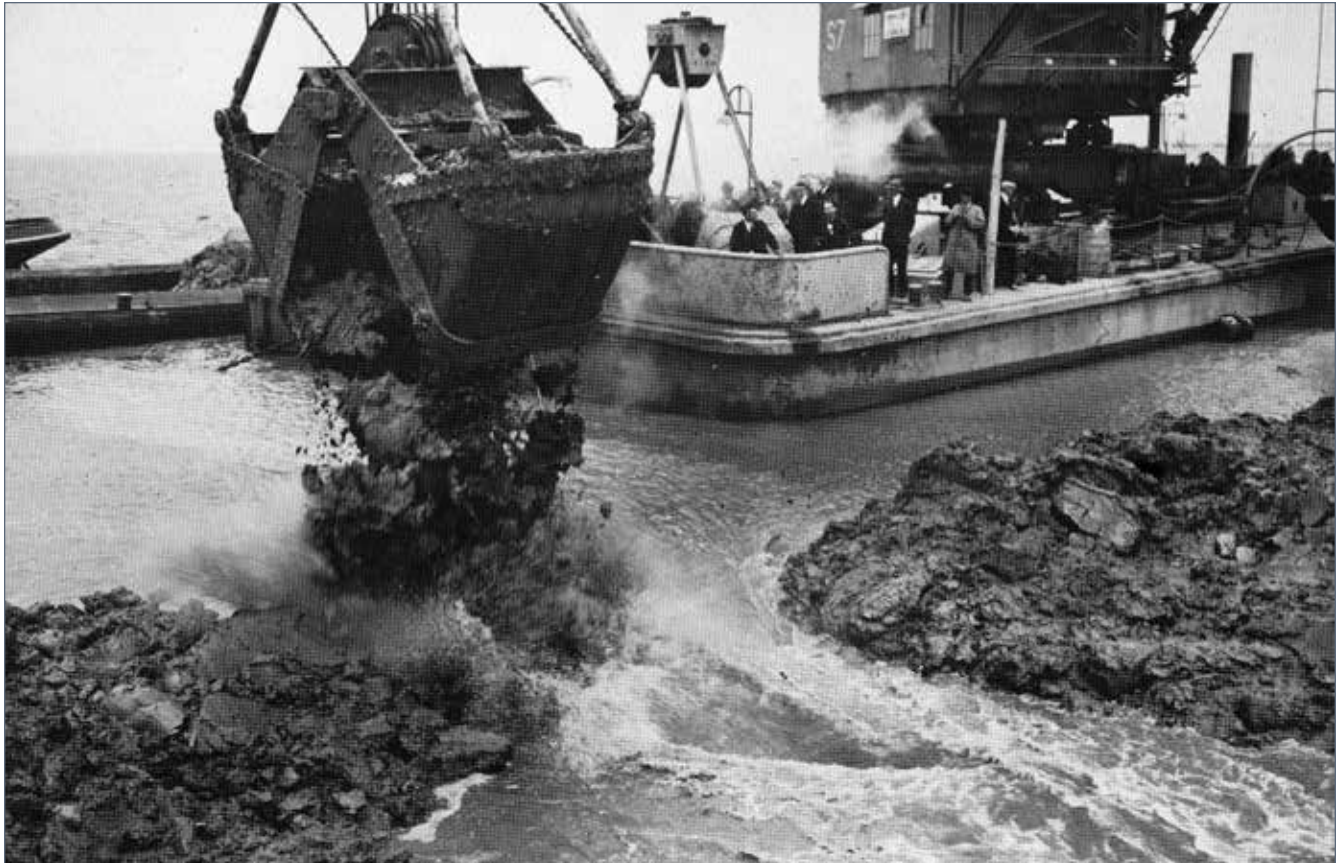
The final gap in the Closure Dam is being closed, May 28, 1932
