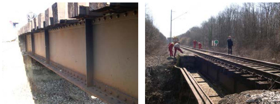
Figure 1 Location of Buna bridge
