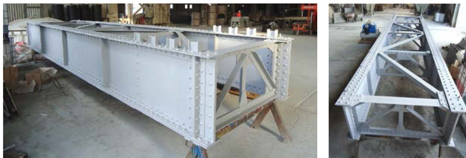
Figure 7 Bridge in process of rehabilitation
