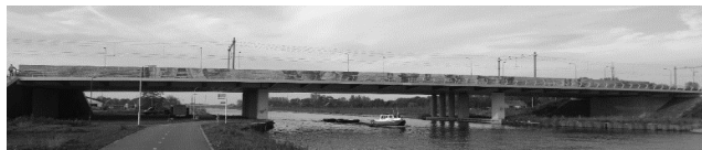
Figure 18. Monitored railway bridge in Rosmalen.
