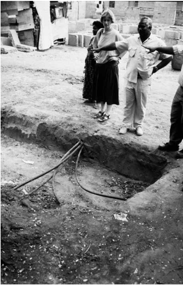
Figure 3.6: Informal and illegal water connections in Dar es Salaam, Tanzania
