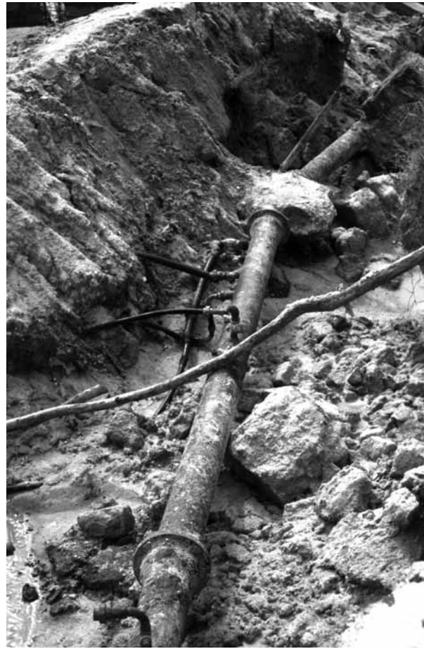
Figure 3.6: Informal and illegal water connections in Dar es Salaam, Tanzania
