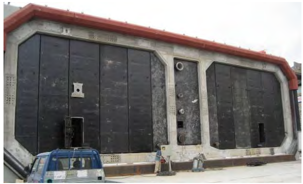
Figure 9. Baseplates on bulkhead
