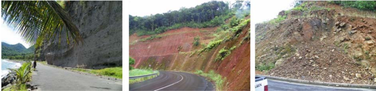
Figure 5-3. Examples of outcrops in volcanic deposits in Dominica. Note the high degree of weathering in the middle photo.
