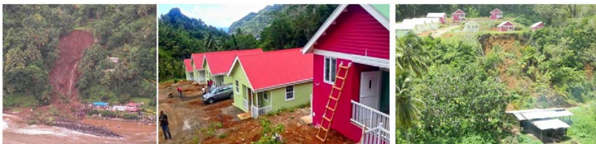
Figure 4-12: San Sauveur landslide which occurred on 24/05/2010 and which killed three people. The government decided to relocate 10 families and with a donation from the Chinese government a resettlement was carried out which was completed in 2015. The area was affected again in August 2015 during tropical storm Erika (right Figure from Garner et al, (2015))
