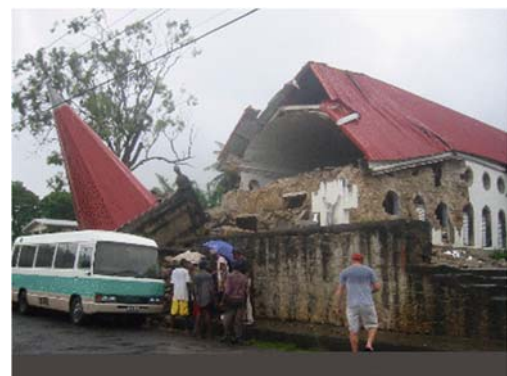
Figure 3-2: Collapsed church tower in Portsmouth caused by the 2004 earthquake.
