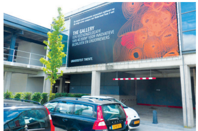
FIGURE 16: A banner at the entrance to the Gallery Car Park
