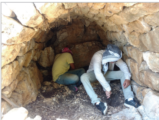
Fig. 36- Cleaning the interior of the arched structure.
