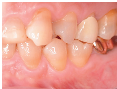
Fig. 11 Temporarily cemented provisional restoration (L5)
