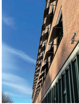
Figure 11.75 Photo of the A-building's exterior screens.
