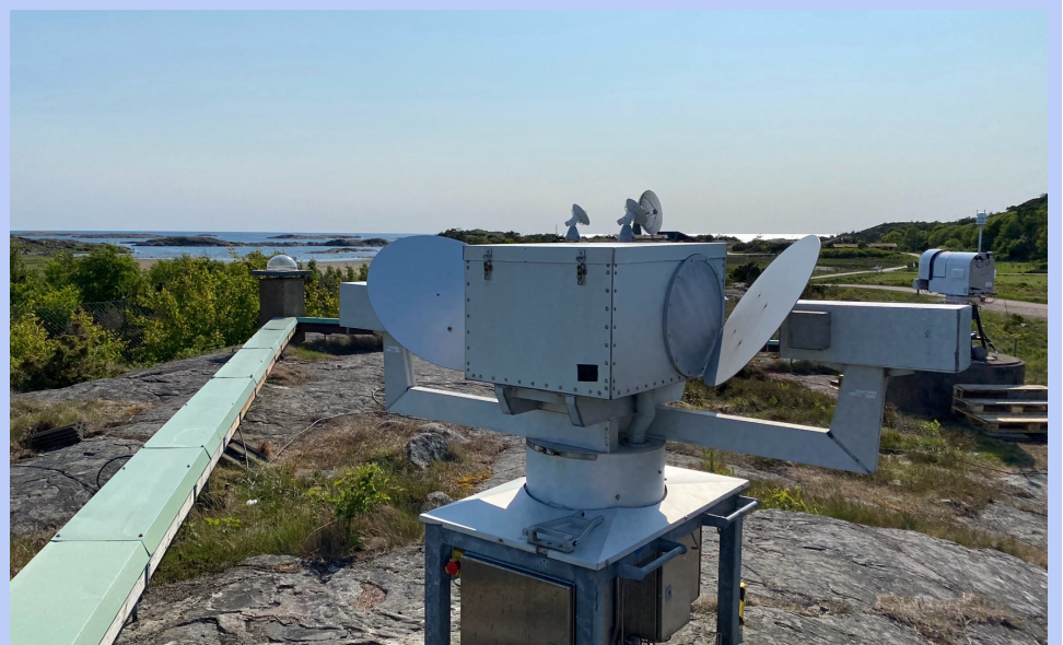
Figure 1. The GNSS station ONSA (left) and the Water Vapour Radiometer (WVR) Konrad (in the foreground). The twin telescopes, and the 25 m radio telescope, are seen in the background. A new WVR (to the right), manufactured by RPG, was installed in May 2023, but has not been used in this study.
